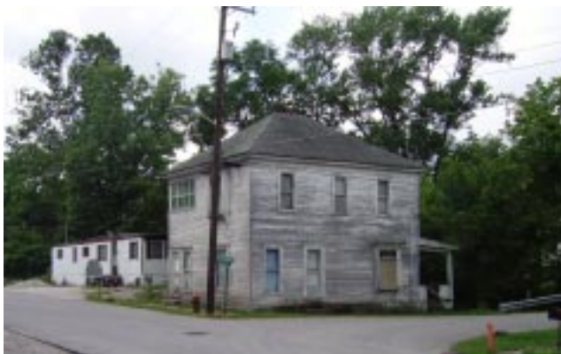
Old structure in Marengo at the corner of Jefferson and Depot streets.
